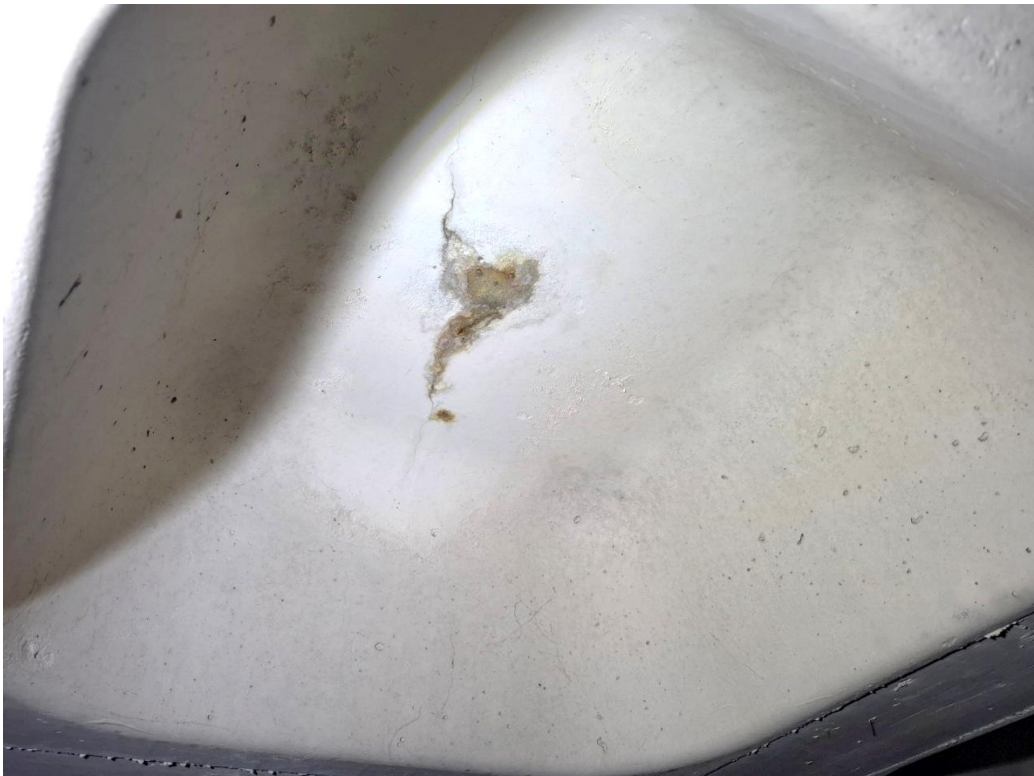
Photograph 2 – local staining from corroding reinforcement
