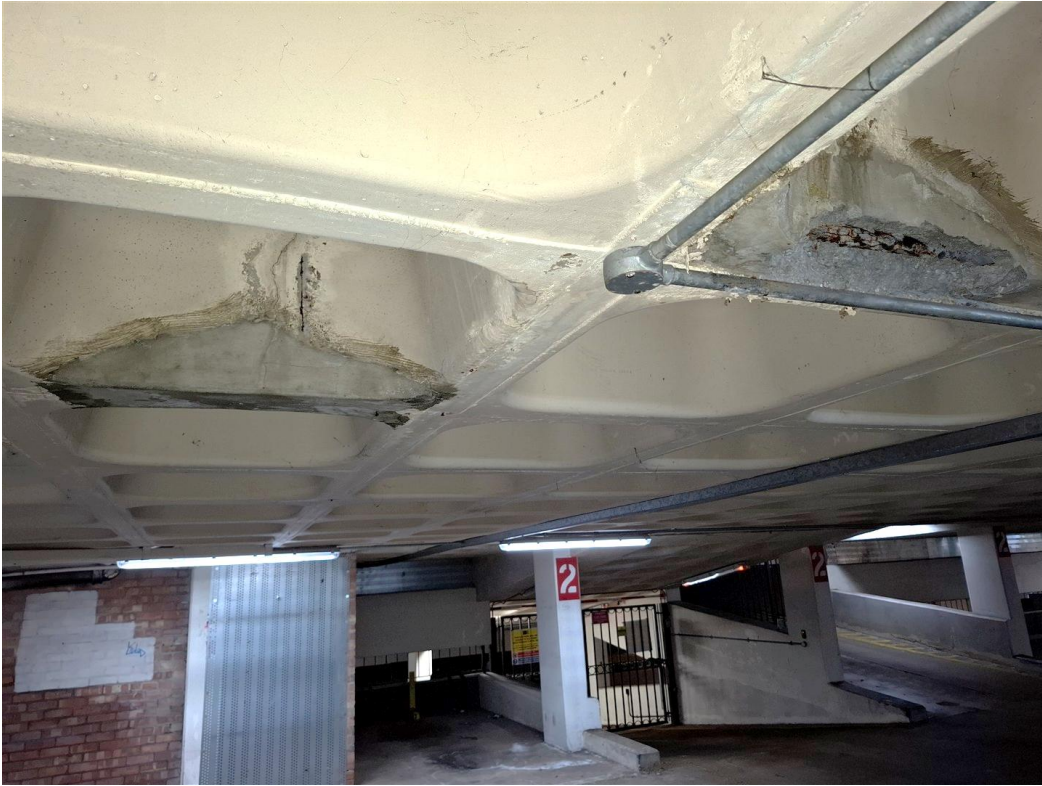
Photograph 2 – local staining from corroding reinforcement
