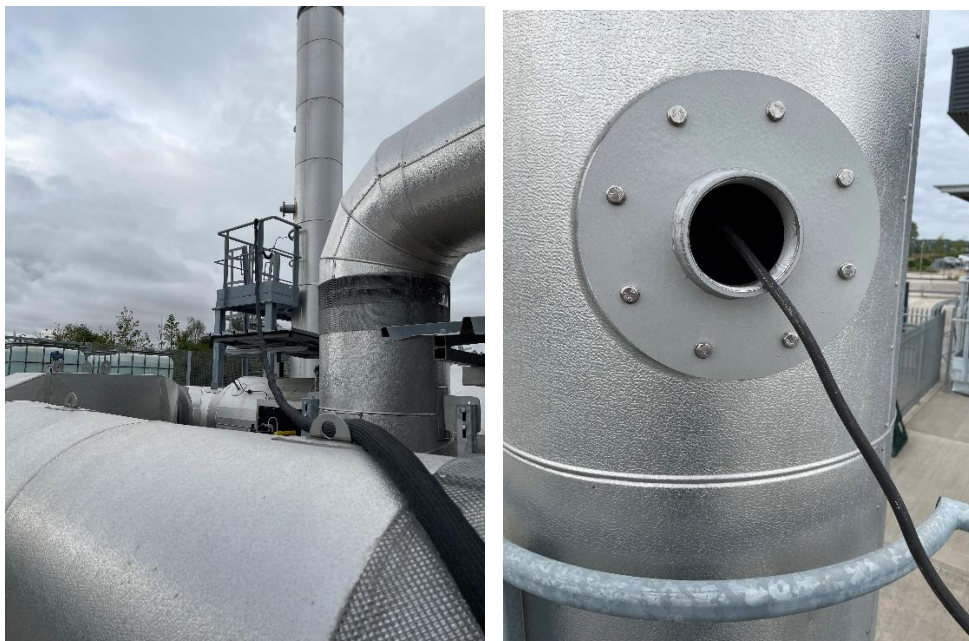
Figure 5: RTO (A2) sample port
