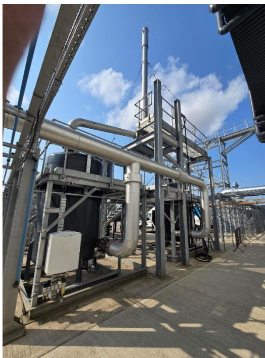
Figure 2: Carbon Scrubber Stack (A1) Monitoring Platform
