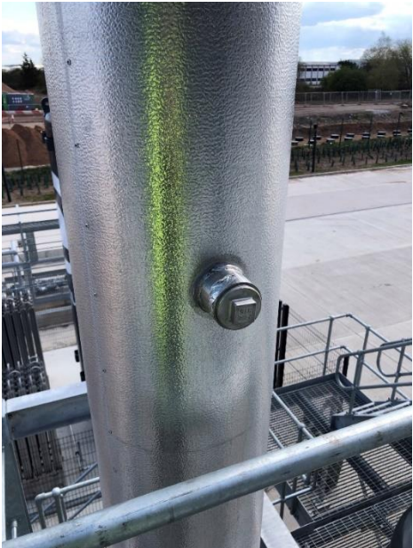
Figure 3: Carbon Scrubber Stack (A1) Sampling Port
