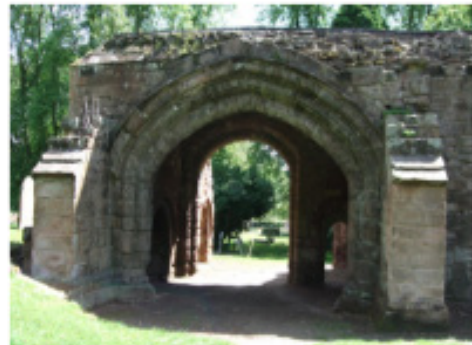
The vaulted passage of the Gatehouse today
