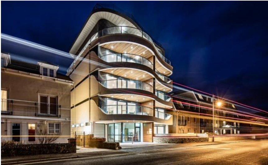
Passivhaus Plus block of flats in Seaton, Devon. Reported an EUI of 25 kWh/m 2 /yr* and solar generation of 18 kWh/m 2 /yr* from 2019-2020.
