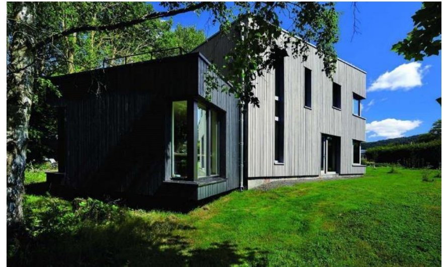
Passivhaus detached house in Worcestershire. Reported an EUI of 27 kWh/m 2 /yr* and solar generation estimated at 19 kWh/m 2 /yr* in 2017.
