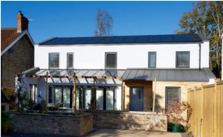
Passivhaus Plus detached home in Bristol. Reported an EUI of 30 kWh/m 2 /yr* and solar generation of 40 kWh/m 2 /yr* from 2019-2020.
