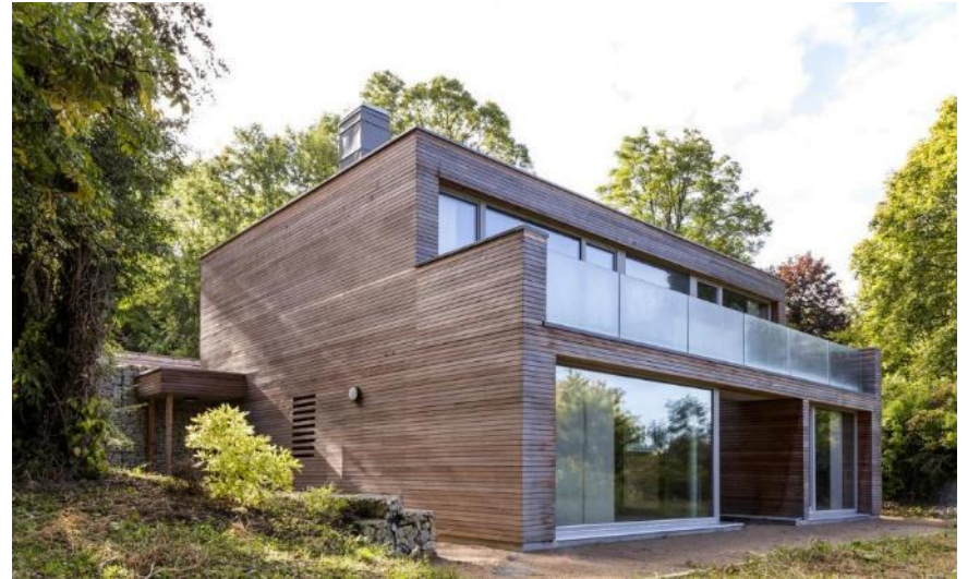
Passivhaus Plus detached house in Buckinghamshire. Reported an EUI of 25 kWh/m 2 /yr* and solar generation of 18 kWh/m 2 /yr* from 2019-2020.
