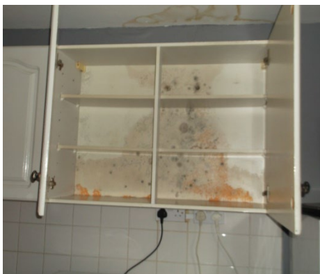
Penetrating damp to kitchen wall and ceiling
