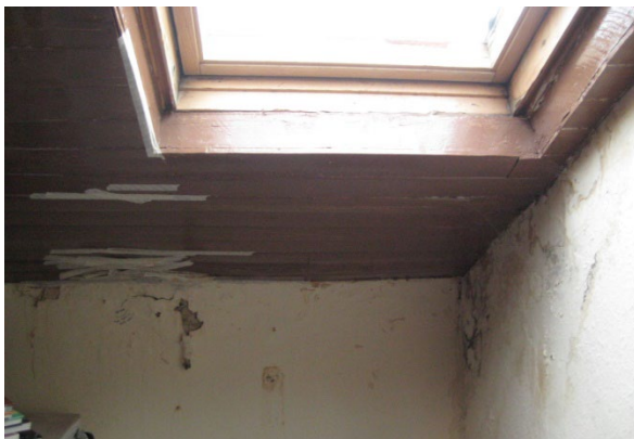
Leaking roof around roof-light in bedroom
