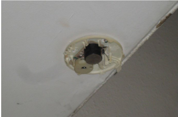
Defective smoke detector
