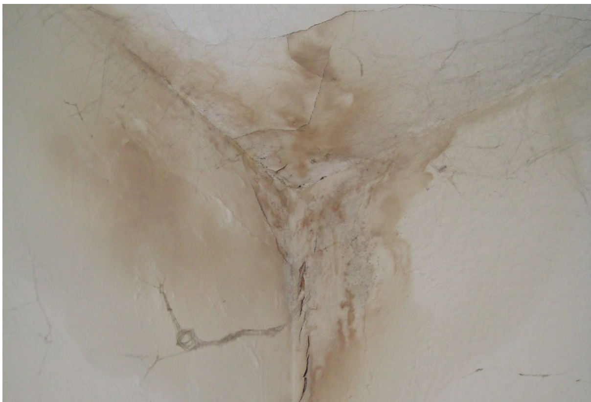
Damp penetration from leaking shower
