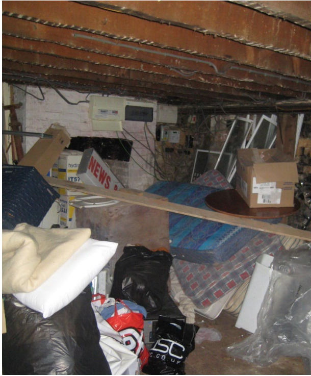
Accumulation of combustible material in cellar
