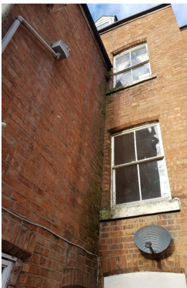
Penetrating damp from defective guttering
