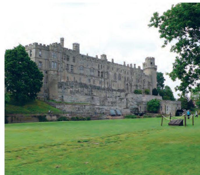
The south front from the Island
