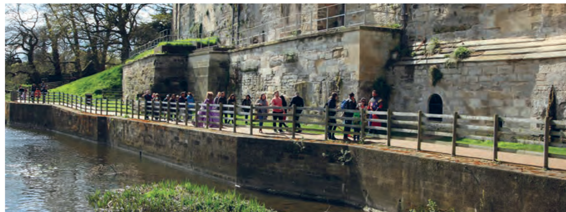
River wall after repairs
