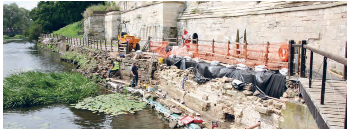
River wall during repairs
