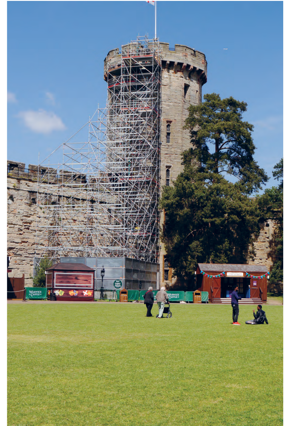
Guy's Tower during repairs
