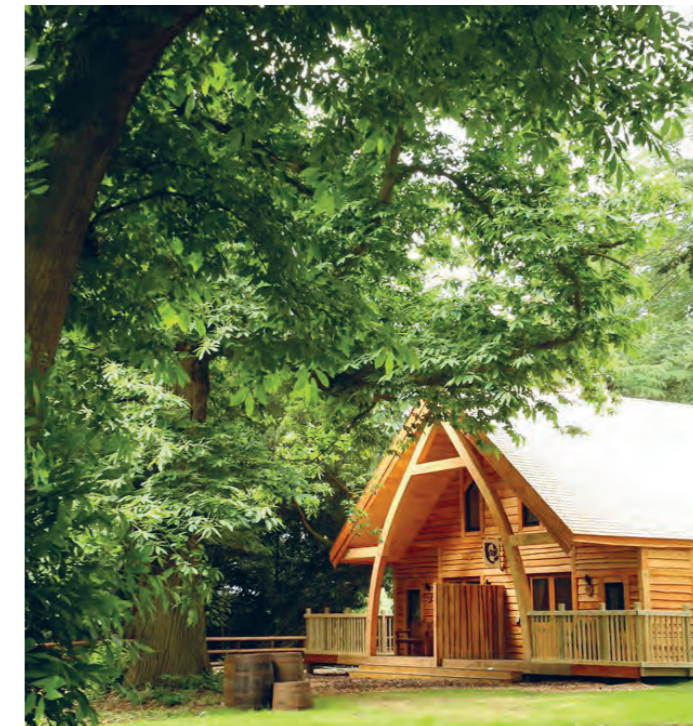
Erection of 14 permanent semi-detached lodges (28 units) for visitor accommodation
