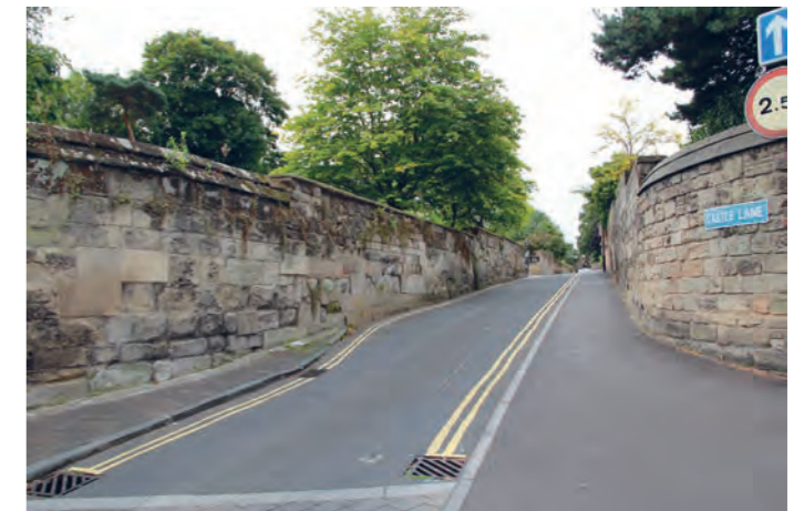
Portion of Boundary Wall to Castle Lane
