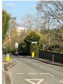
9 - Cromwell Lane Bridge
