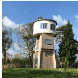
24 - Water Tower Hob Lane
