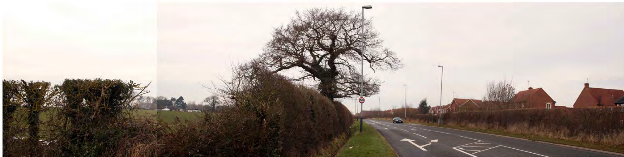
View E2 - looking north-west on Harbury Lane. Housing at Warwick Gates on the right and 'Heathcote Park' (mobile homes) are just visible through the hedge on the left.
