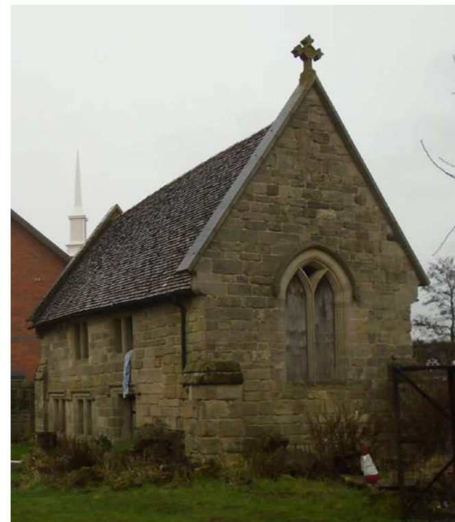
Current photo of St Michael's Chapel, north and west elevations
