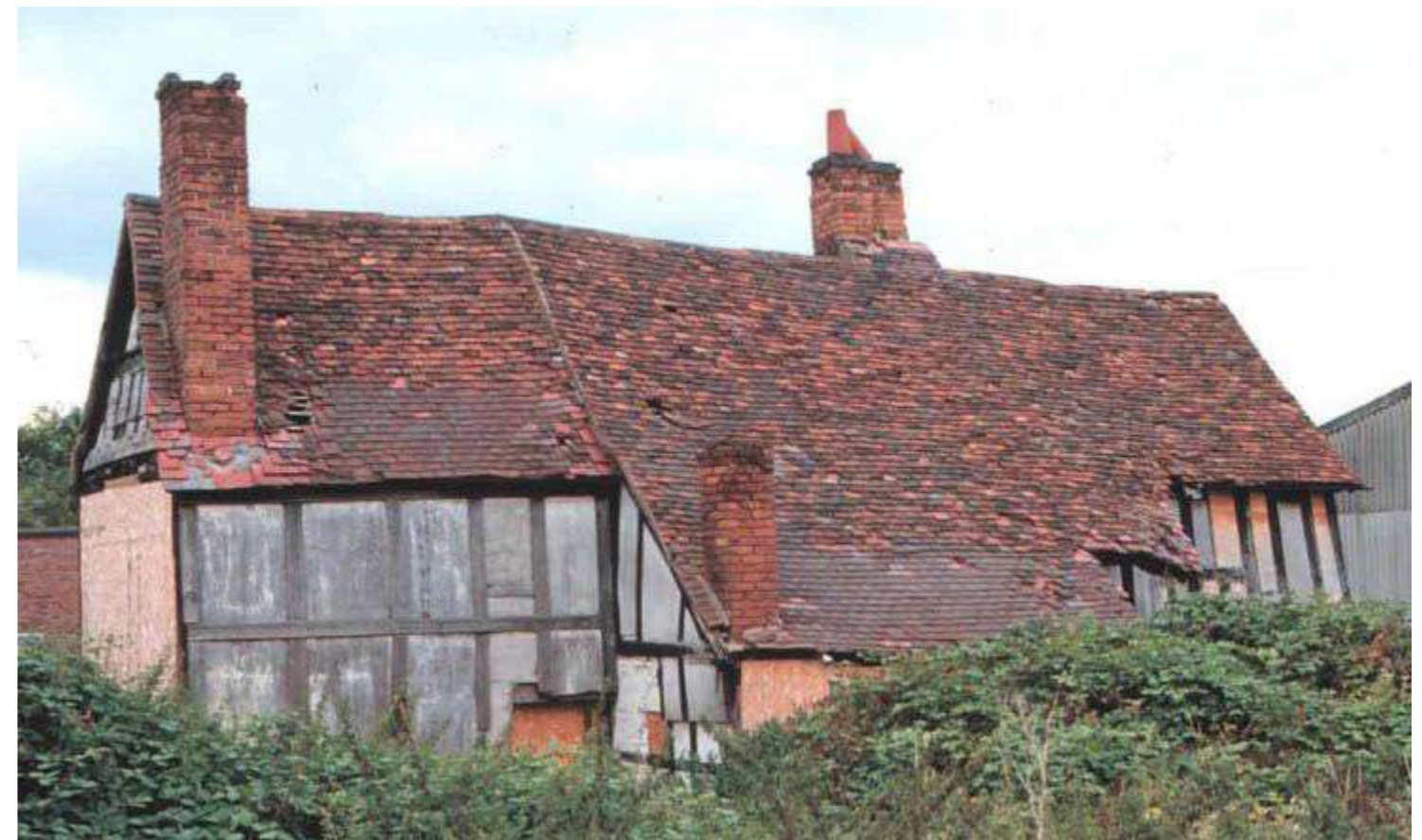
View of the south west elevation of Master's House c 1990s
