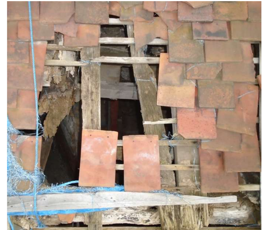
Existing Tiles on the Master's House
