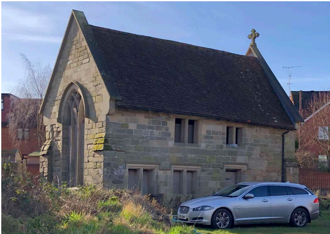
Photo of the north elevation of St Michael's Chapel c 2020 showing new stonework and tiled roof
