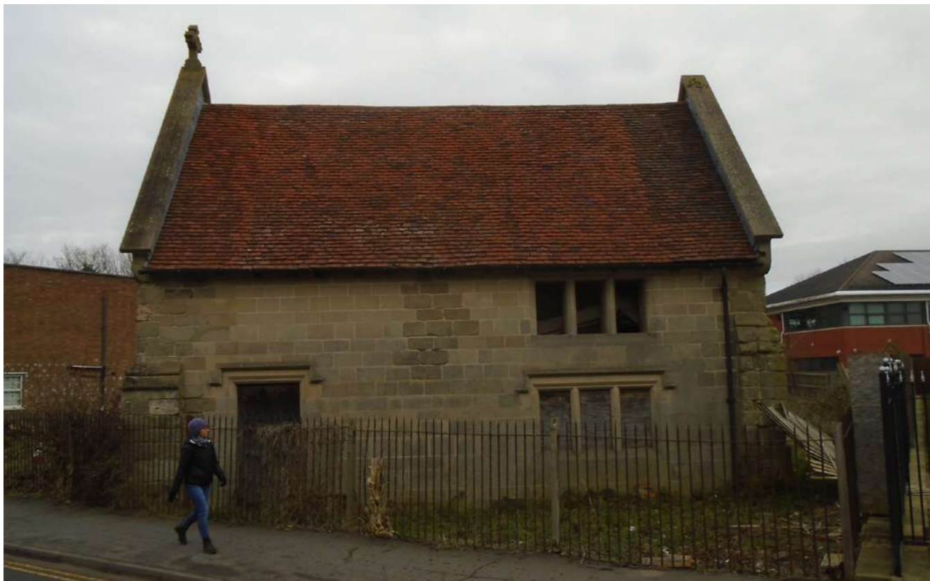
Photo of St Michael's Chapel c 2020, showing new stonework and tiled roof
