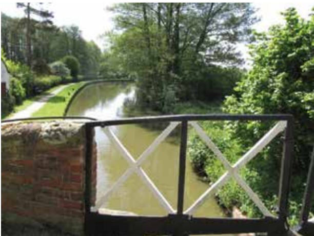
The canal at Lowsonford (WDC)
