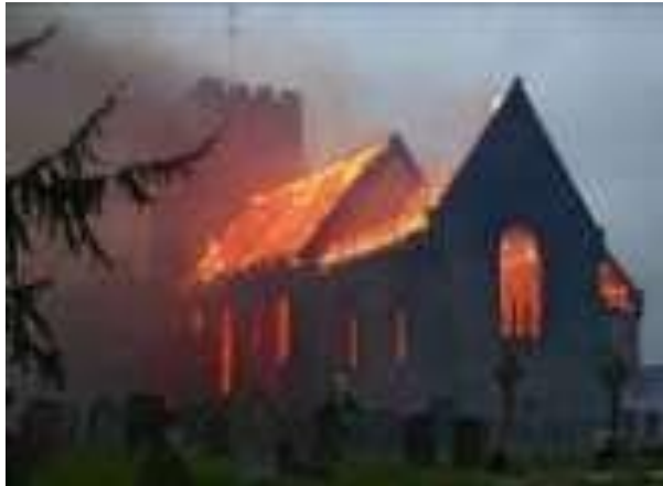
Figure 3 St Nicholas Church fire, 2008
