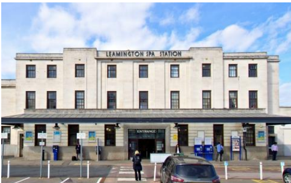
2 Leamington Spa Railway station (David Heathfield)
