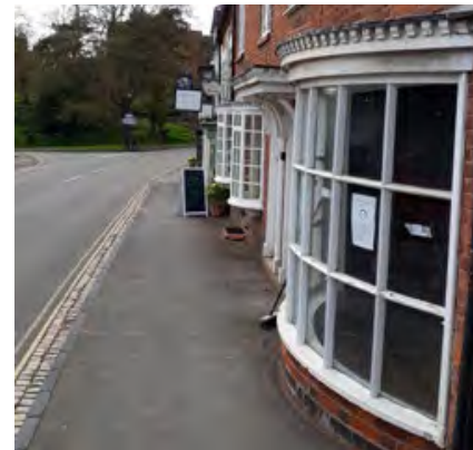
Bow bay windows provide a dominant architectural feature
