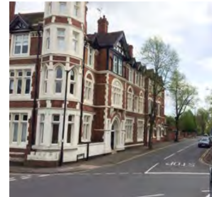
Large building plot with distinctive architecture helping to define the junction to Abbey Hill and create a sense of arrival.
