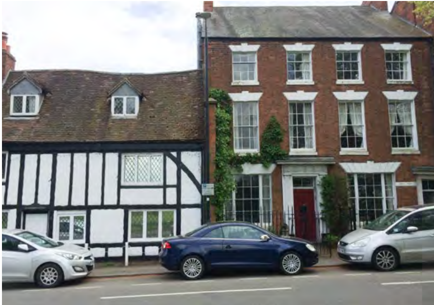
3 and 4 storey properties facing onto Abbey Hill
