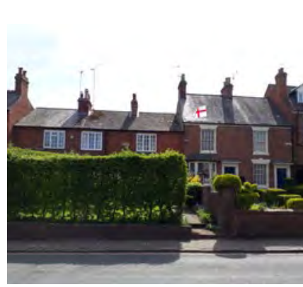
Road incline provides a varied roofscape
