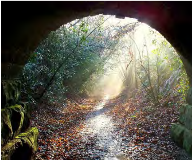
Bridge over Rocky Lane
