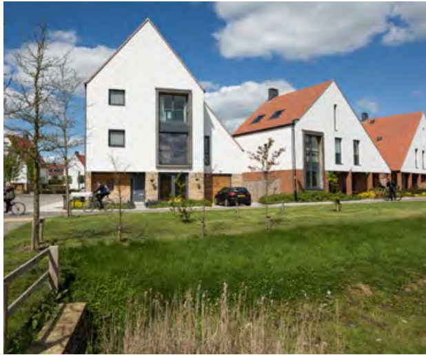
Housing adjacent to a lane and SUDS system
