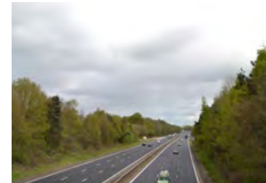
A46 - Six lane dual carriageway
