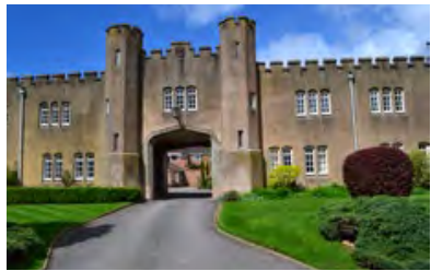
Stables at Thickthorn - Grade II Listed Building
