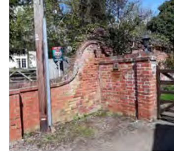
Brick wall with coping and detail
