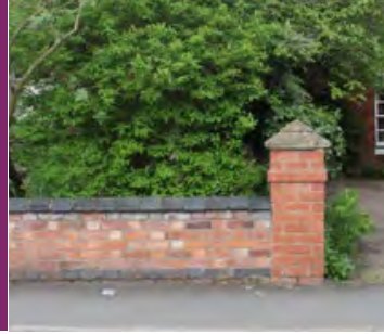
Low brick wall with brick pillars and blue clay tile coping's
