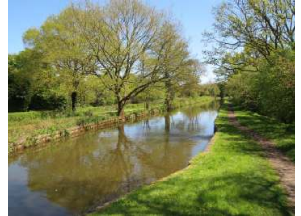
Below the lock the waterway wall on both sides is concrete piling, in some places with substantial tree growth out of it. As this is above the roadway edging will need renewing to keep the water in and be treated in a sensitive manner.
