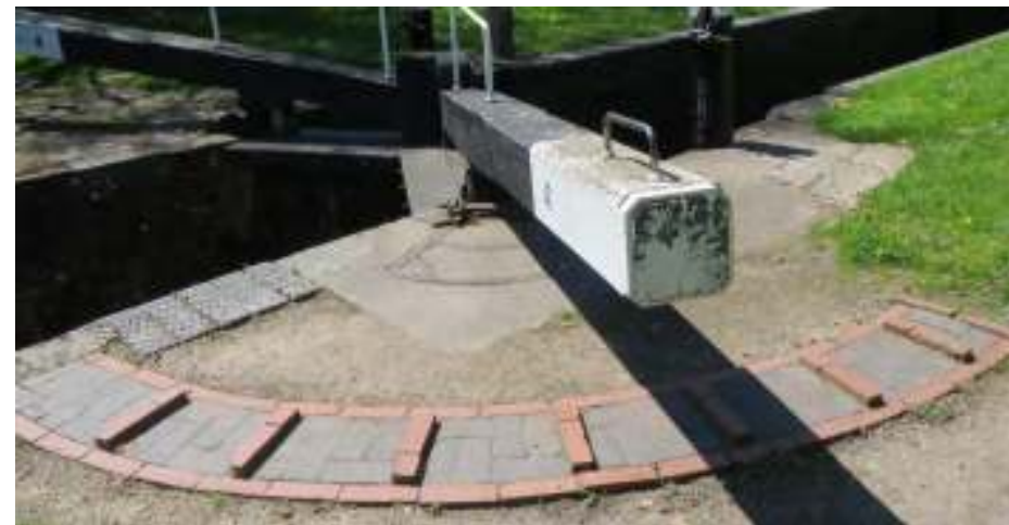
Lock 4 has brick copings and the heelgrip quadrants are in poor condition.
