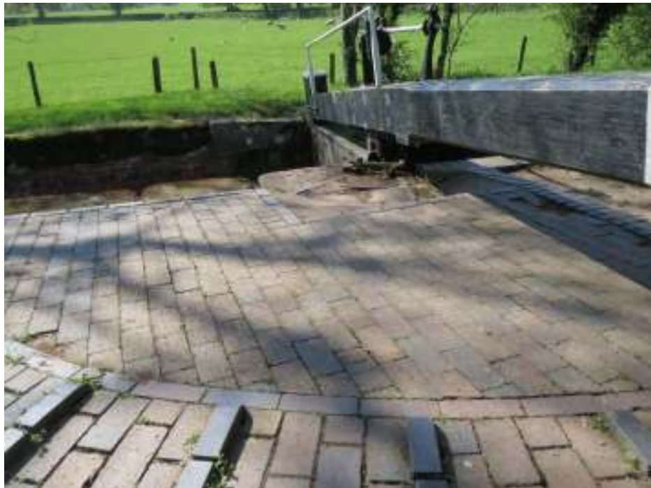
Lock 24 – the heel quadrants are well built but feel imposed as they sit above the level of the coping. Some of the first restoration work has been replaced during the National Trust's stewardship, whilst more recent work was done by British Waterways and follows patterns used nationally. The Canal & River Trust are anxious to ensure that work carried out is researched and seeks to reinforce local distinctiveness.
