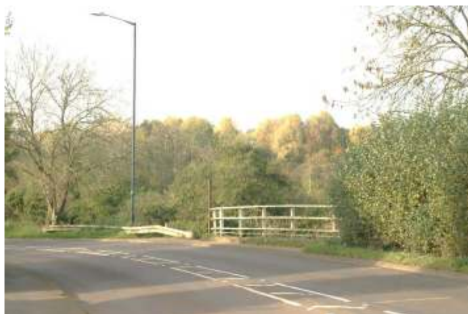
ELEVATED ROADWAY HAS SMOOTHED OUT BRIDGE OVER THE CANAL AND A STEEL ROAD PARAPET IS INTRODUCED.
