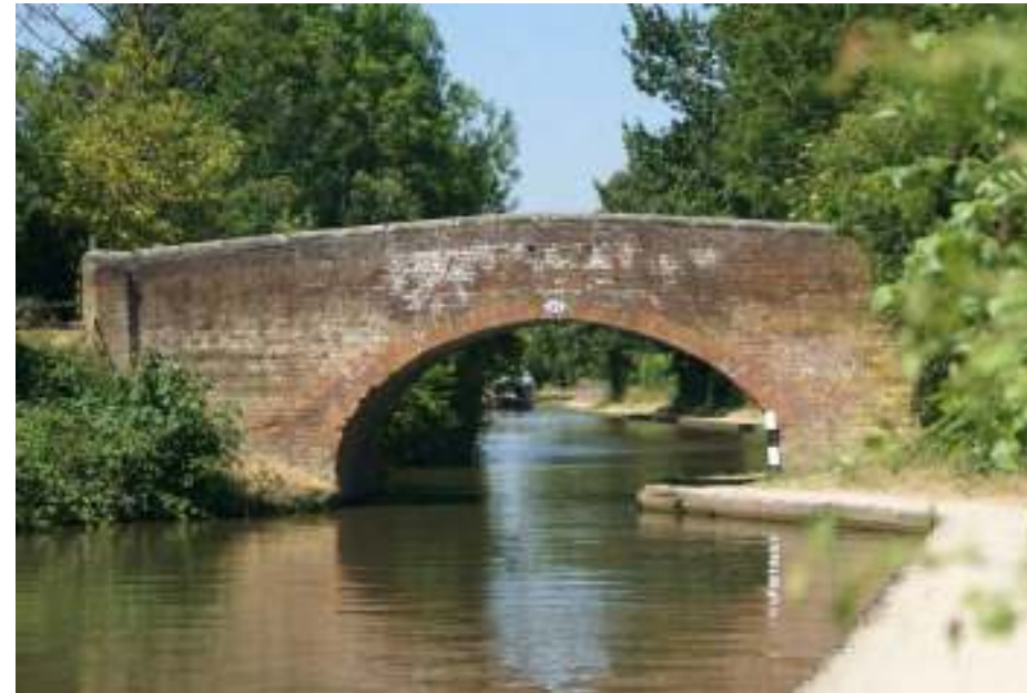
BRICKS WERE DUG AND BAKED LOCALLY TO FORM THESE SIMPLE BRIDGES THAT SPAN THE CANAL AND TOWPATH. RUBBING STRAKE AT ABUTMENT PREVENTS GRIT IN TOW ROPE FROM ERODING BRICK ARRIS
