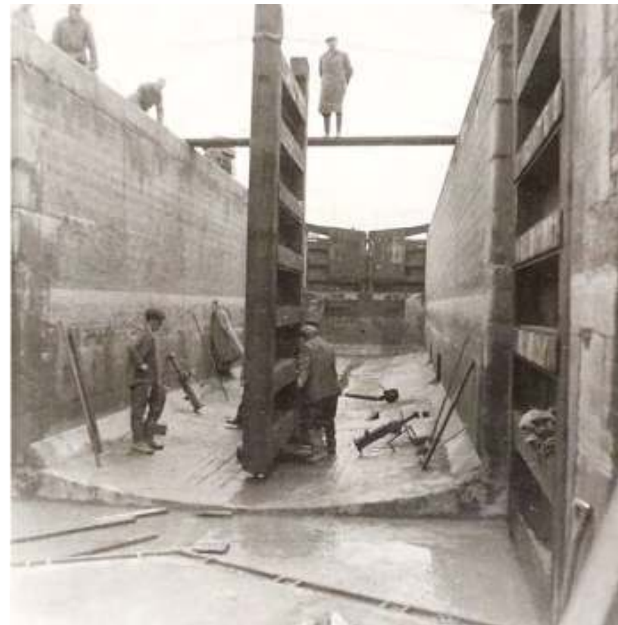
NEW LOCKGATE BEING FITTED IN BROAD LOCK 1958
