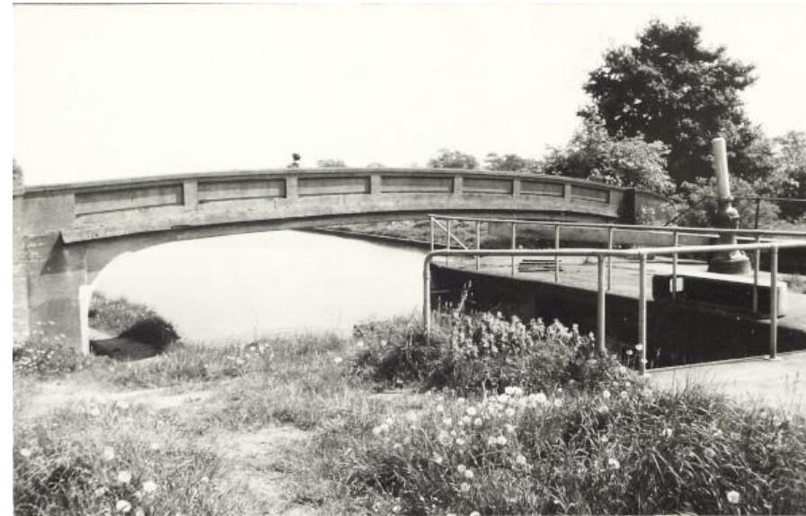
REINFORCED CONCRETE REPLACEMENT BRIDGE BW200
