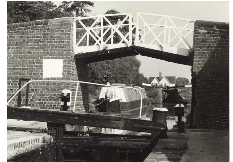
CANTILEVERED SPLIT BRIDGES
