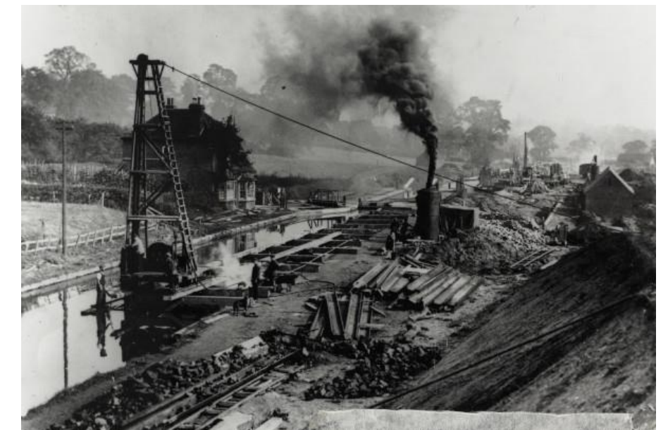
TOP OF HATTON FLIGHT UNDER CONSTRUCTION BW200
