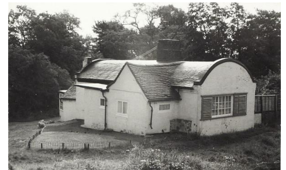
UNIQUE LOCK COTTAGE CONSTRUCTION
