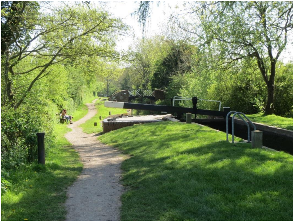
Lock 23 is a turf sided lock chamber with red brick and stone copings and single gates top and bottom There are views out in both directions and listed
