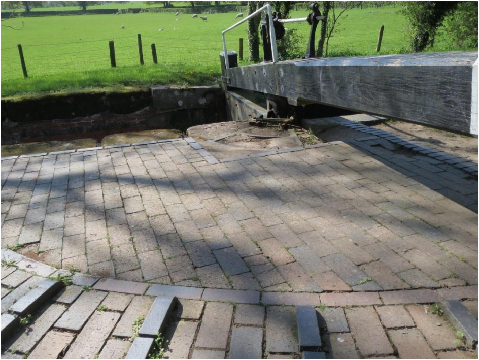
Lock 24 – the heel quadrants are well built but feel imposed as they sit above the level of the coping. Some of the first restoration work has been replace during the National Trusts stewardship, whilst more recent work was done by British Waterways and follows patterns used nationally. The Canal & River Trust are anxious to ensure that work carried out is researched and seeks to reinforce local distinctiveness.
