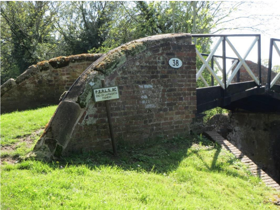
Bridge 38 is a traditional split bridge with metal deck topped with gravel. This is listed as a good example.
