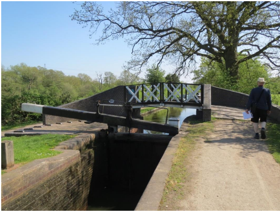
Lock 22 has had a heavy engineered bridge in the style of a split bridge added to take the towpath to east side of the canal, set in very blue brick abutments with sloping brick paving.
