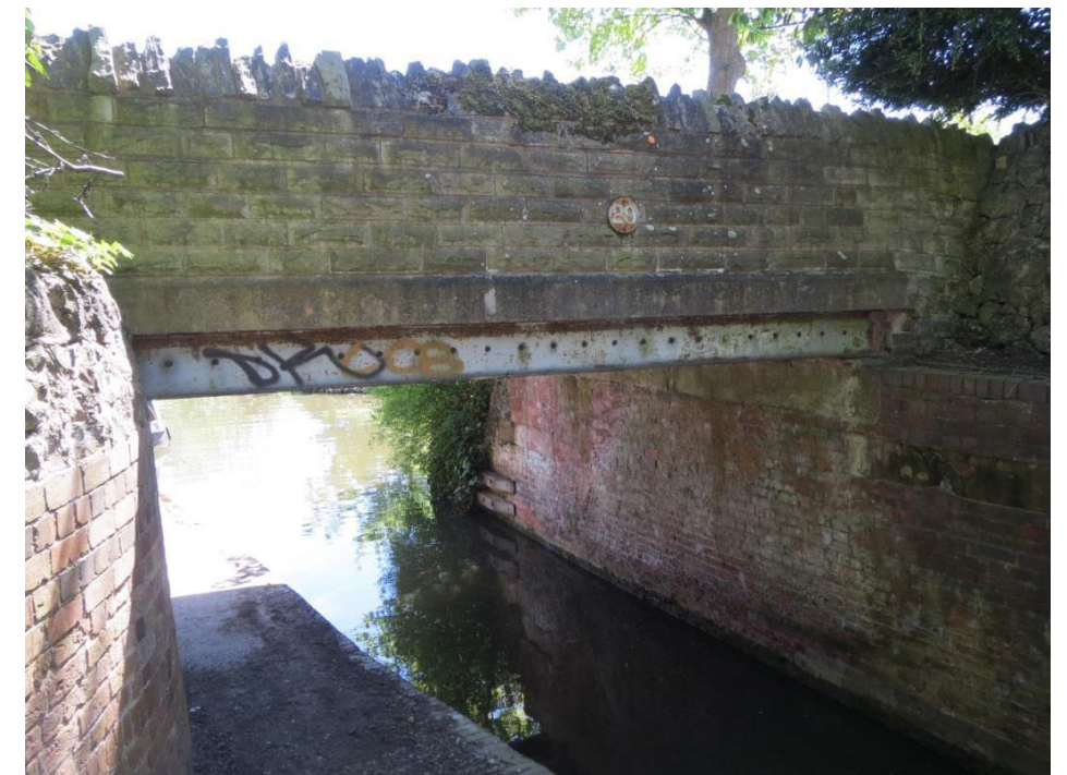
Church Lane connects the canal to the historic core of Lapworth and the fine church. The bridge itself has had a 1920's style stone parapet added above the metal beam.
