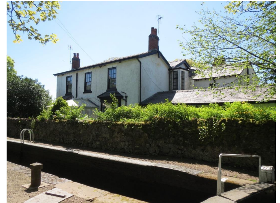
Lapworth top lock, lock no 2 on the canal, is 10 miles from the guillotine lock at Kings Norton, with a single top gate and a pair at the bottom. There are stone copings to the lock chamber with blue diamond brick copings on both the offside and towpath side. Access to the towpath is by the CRT compound, just west of the lock itself.
