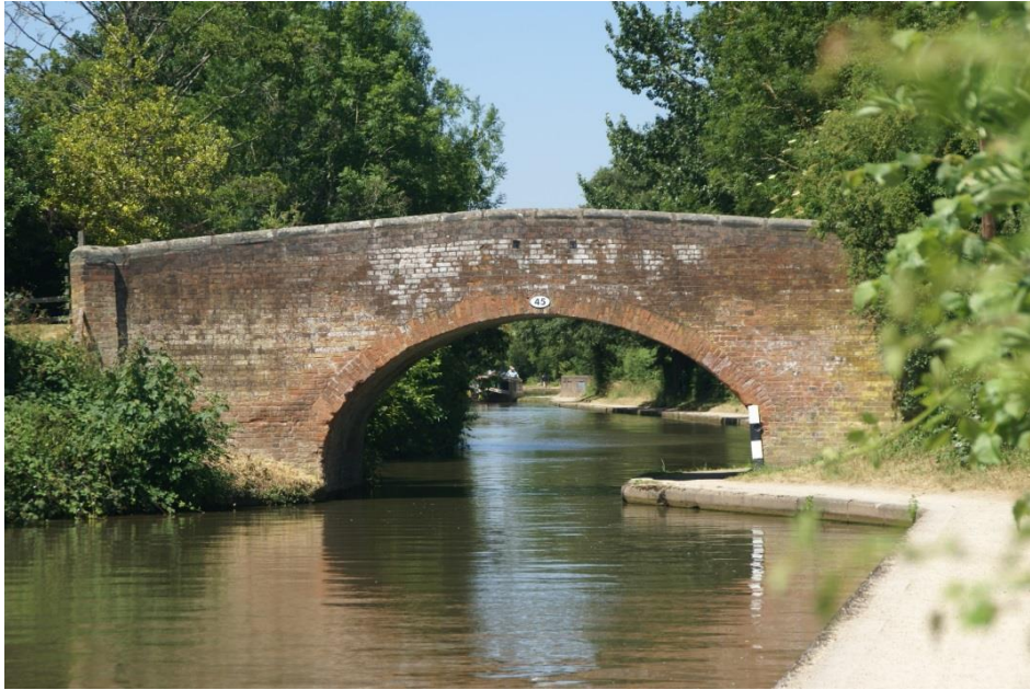
BRICKS WERE DUG AND BAKED KLOCALLY TO FORM THESE SIMPLE BRIDGES THAT SPAN THE CANAL AND TOWPATH. RUBBUING STRAKE AT ABUTMENT PREVENTS GRIT IN TOW ROPE FROM ERODING BRICK ARRIS
