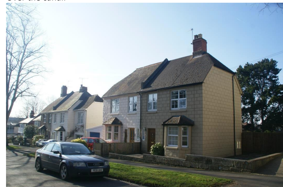
NELSON'S EXPERIMENTAL CAST STONE BLOCKS USED FOR MODEL WORKERS DWELLINGS.
