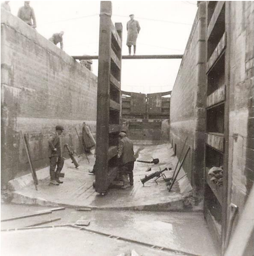
NEWLOCKGATE BEING FITTED IN BROAD LOCK BW1958
