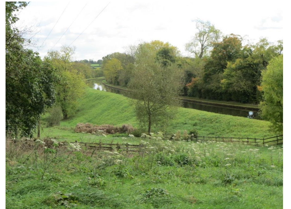
Rowington cutting is followed by a grand embankment that enlarges the setting again. The spoil from the cutting was barrowed to make the bank,.
