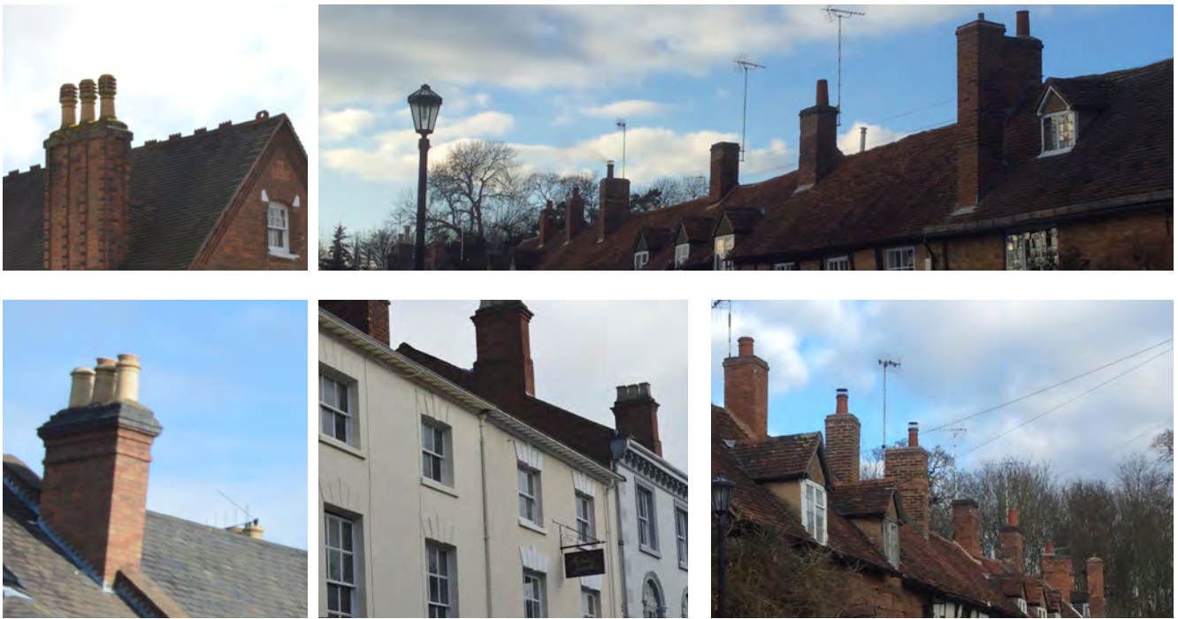
Characterful Chimneys; regularly used to bring roof line variation to the streetscene
