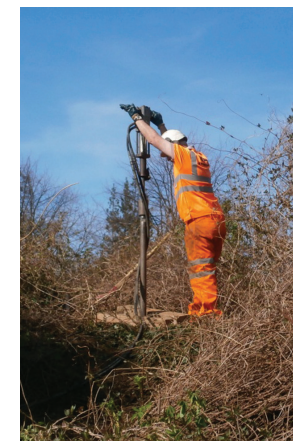
In difficult-to-access locations, hand-held equipment can be used. Image courtesy of CH2M Hill.
