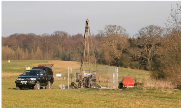
Cable percussion borehole. Image courtesy of CH 2 M Hill.
