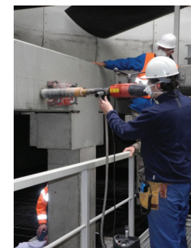
Concrete core (structural investigation). Image courtesy of CH2M Hill.
