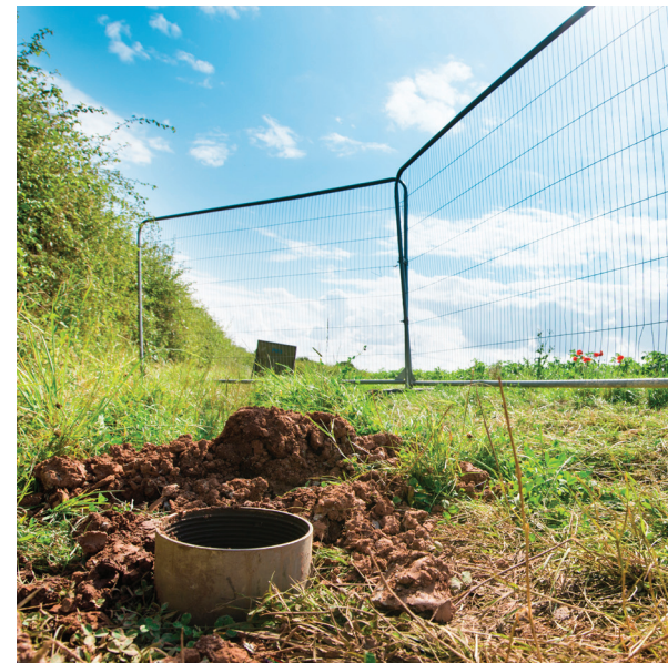
On completion, boreholes are filled or further instrumentation installed. Image: HS 2 Ltd.
