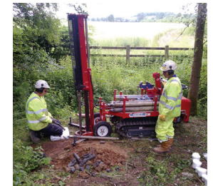
A motor-driven hammer pushes a cone into the ground for dynamic probing. Image courtesy of CH2M Hill.
