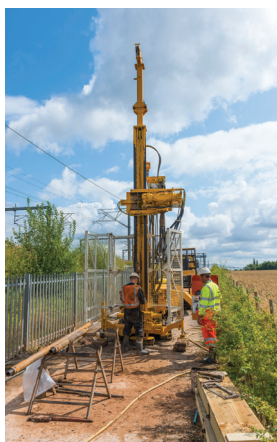
Drilling of a small borehole via a rotary core rig. Image: HS2 Ltd.
