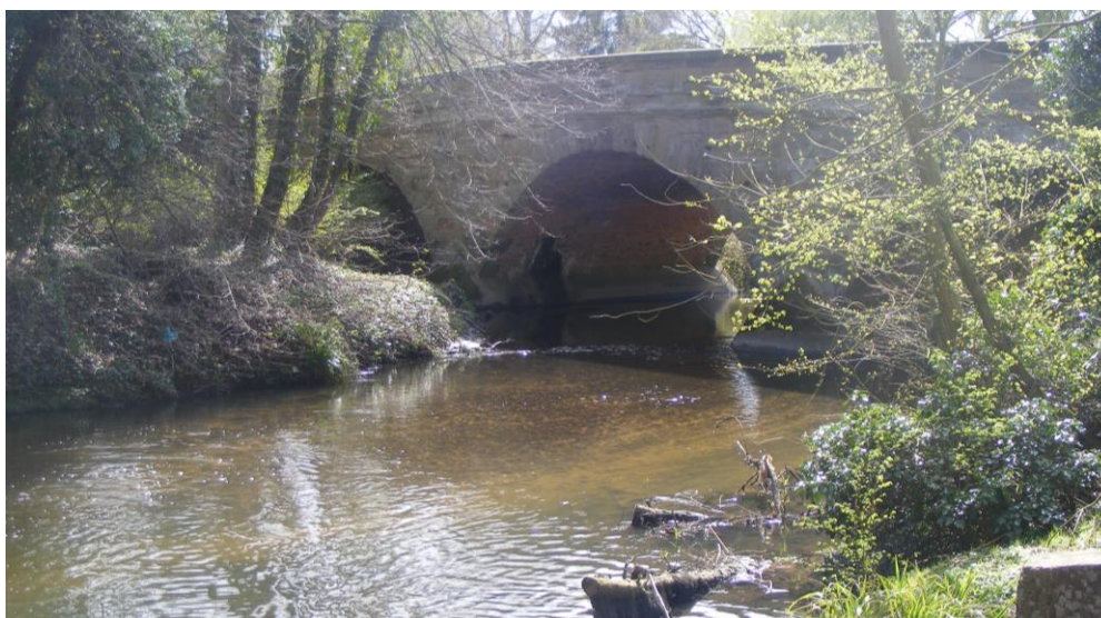
River Sowe, Baginton Bridge
