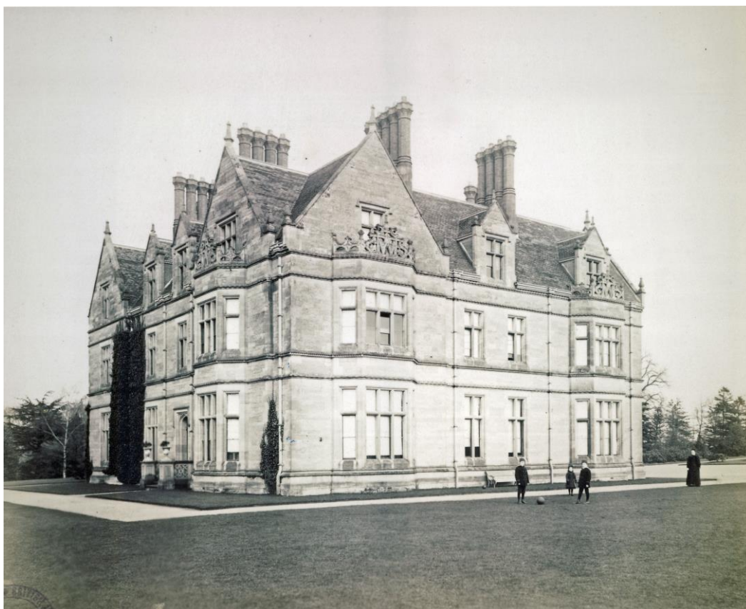
Woodcote c.1891 showing south and west fronts
