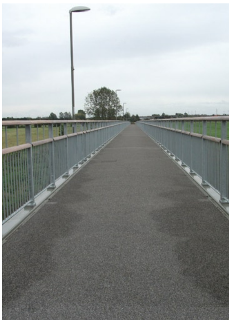
Lighting columns positioned outside bridge parapet to maximise effective width, St Neots
