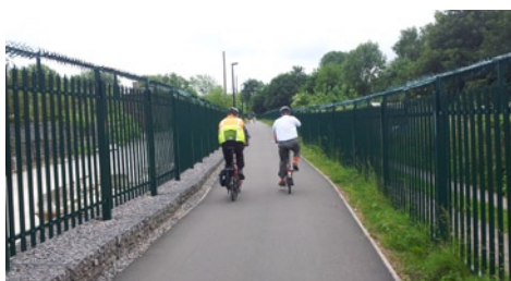
Bristol – Fencing and signing set back beyond the path edge to maximise effective width
