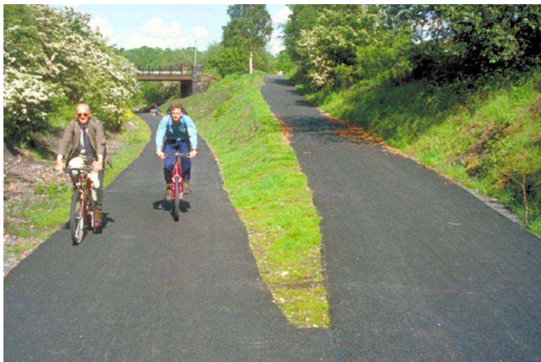
View of a railway path cutting in Paisley showing a long, evenly graded and gentle ramp connecting with an access point. Notice how the ramp has been constructed with fill brought in, but still leaving space for the main path to continue on the level. But because the path level itself has not changed, the ramp is very long (as is the one in the other direction, just under the bridge in the distance)
