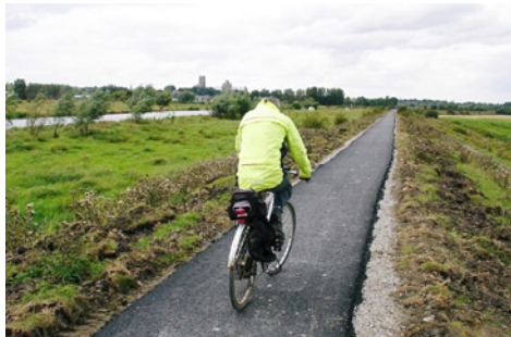
Flood bank, River Ouse, Ely, Cambs
