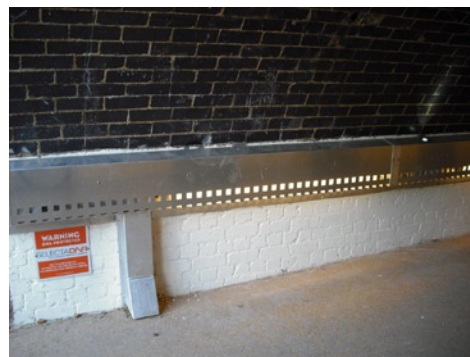
Vandal proof lighting units, Dartford
