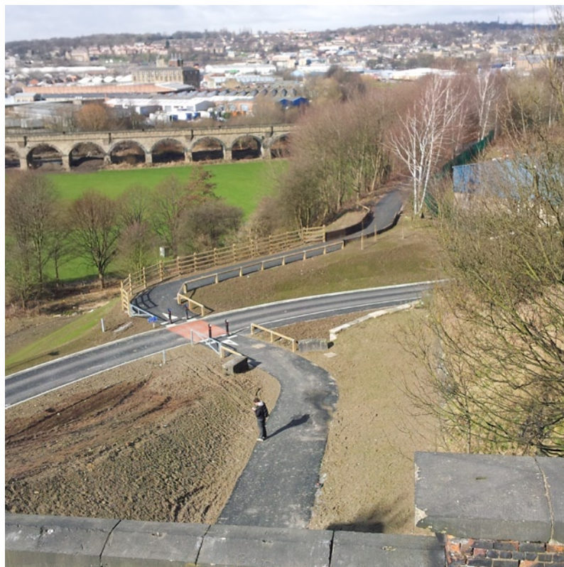
Radius introduced to slow cyclists at a minor road crossing, Dewsbury
