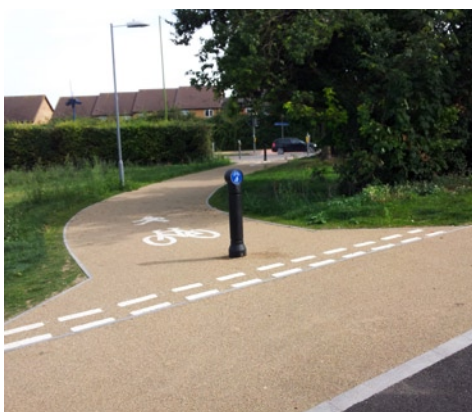
45° chamfer at intersection, Royston
