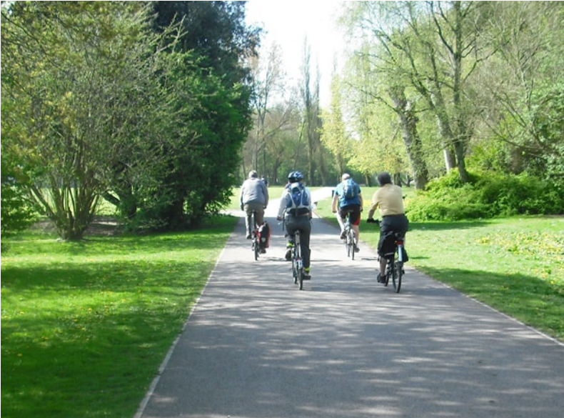
Southampton –width enables cyclists to overtake each other and pass oncoming cyclists simultaneously – a requirement on busy commuter routes
