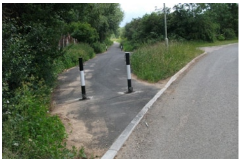
Re-use of old road, Meadow Lane, Syston
