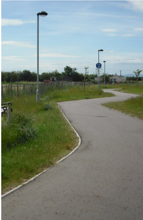
Lighting columns positioned outside path margin to maximise effective width, Ballymoney
