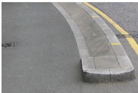
Use of shallow angled battered kerb to increase effective width, London
