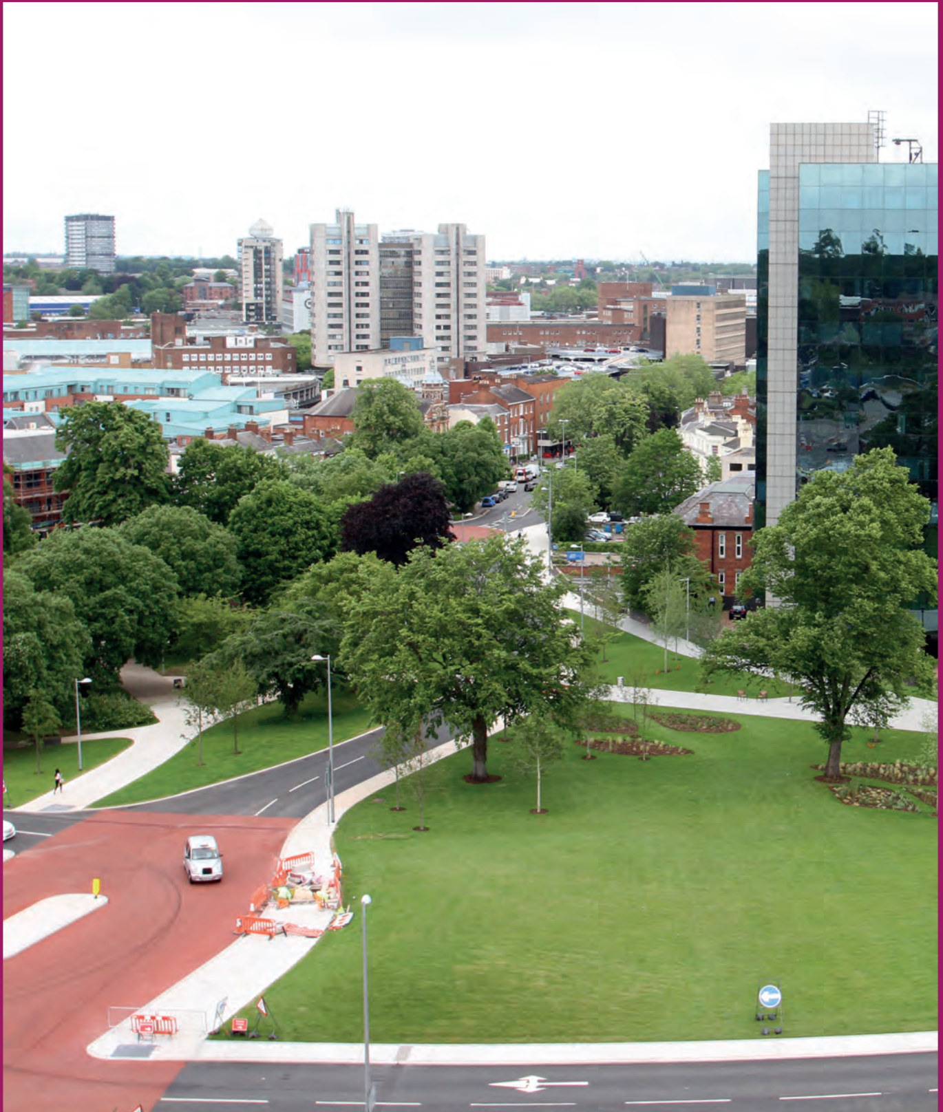
Ring Road Junction 6
