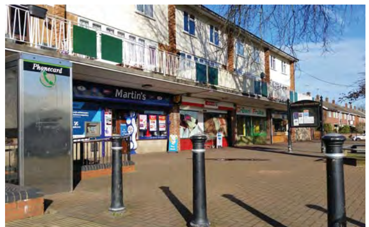
Crown Way Local Centre having accommodation above
