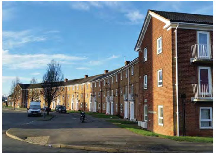
Strong block form/focal building on Newland Road
