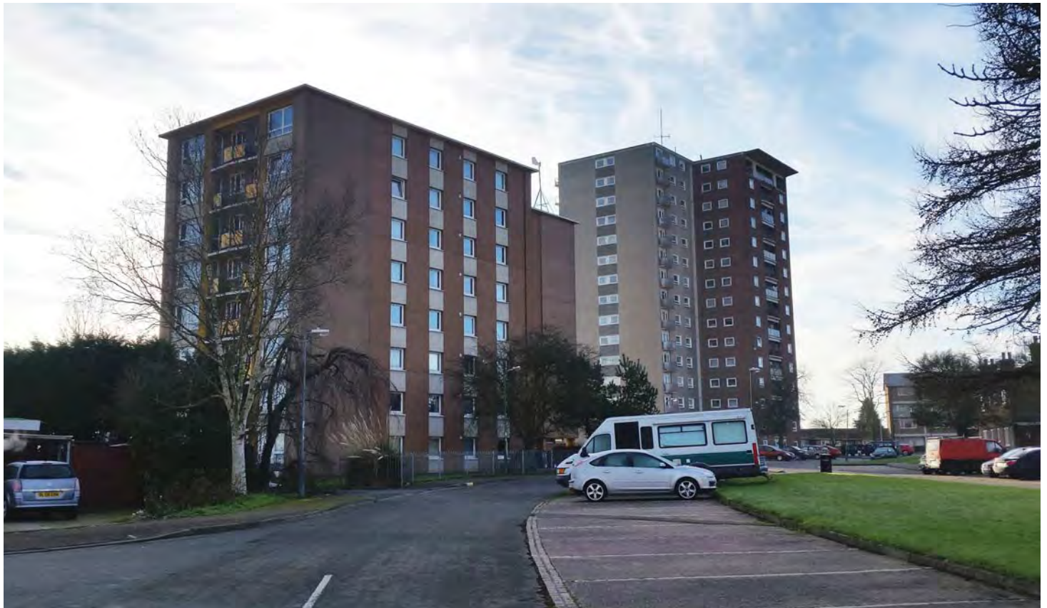
High-rise accommodation directly north of the Site at The Crest. Subject to the Council's regeneration proposals.
