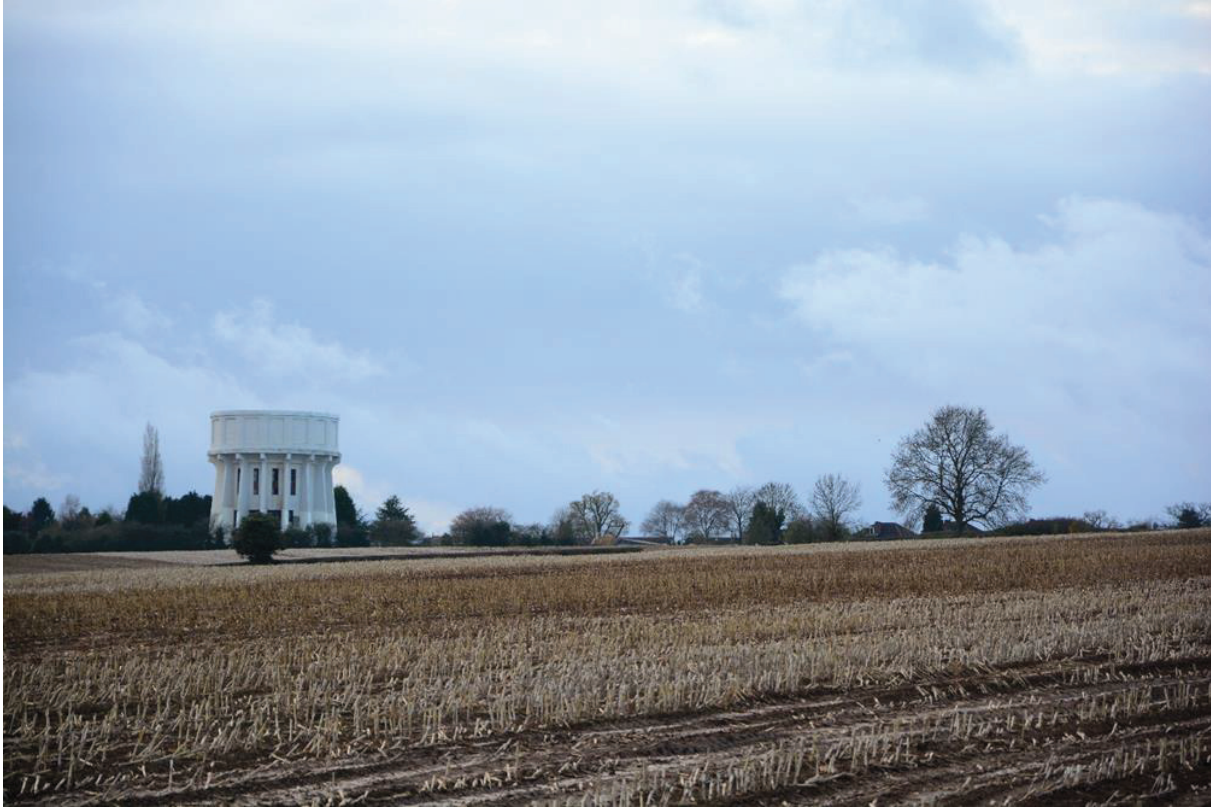
Photo 1: Early 20th century water tower on western boundary of (SHLAA C02, C03, C13; C23)
