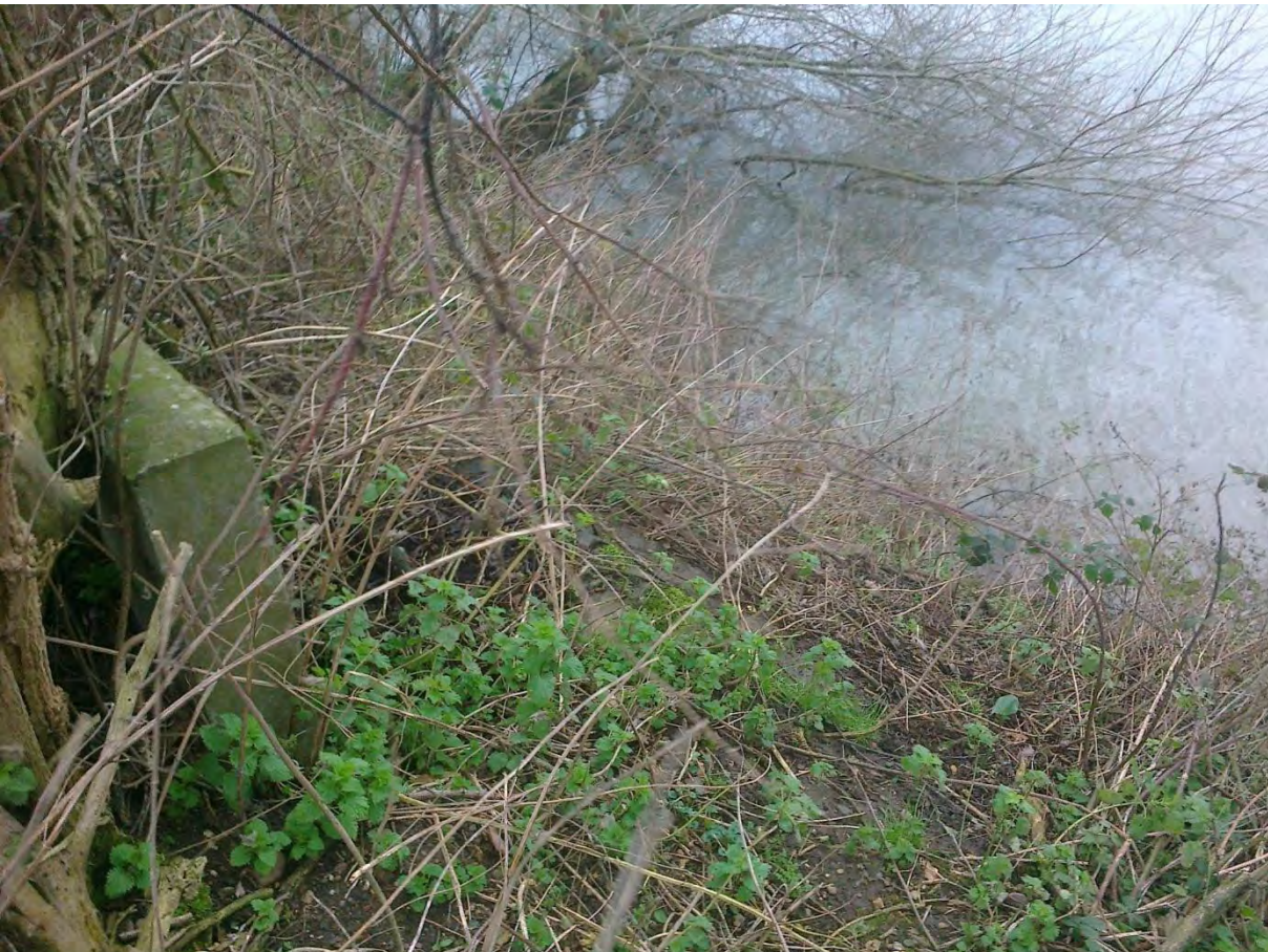
Photo 14 – Headwall near south end Severn Trent Water compound discharging to River Avon.
