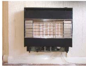
Gas fire and back boiler
