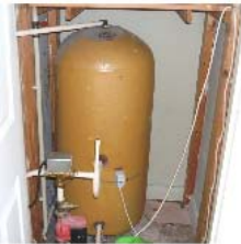
Hot water cylinder with thermostat
