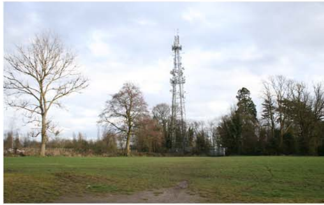
Mast in south-east corner of site. Note also the mature trees along south and east boundaries.
