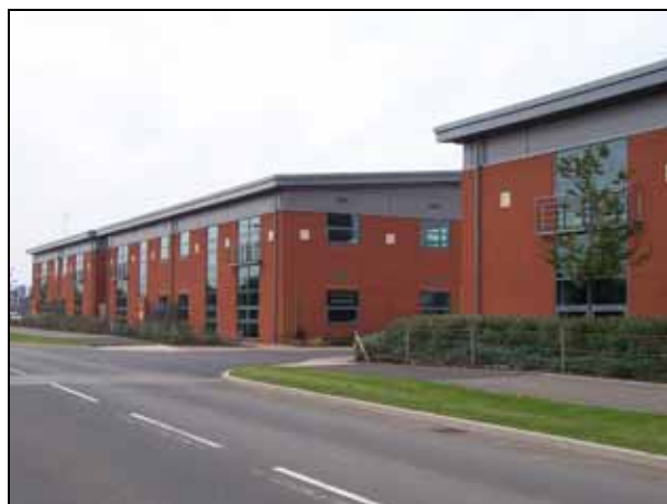
Completed Office Development at South West Warwick.
