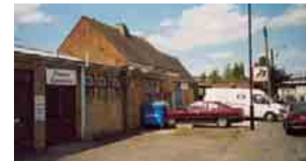
The Council leases Milverton House
