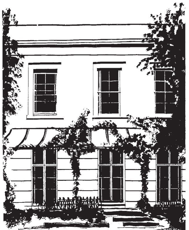
A typical Regency property with original windows and french casements.
