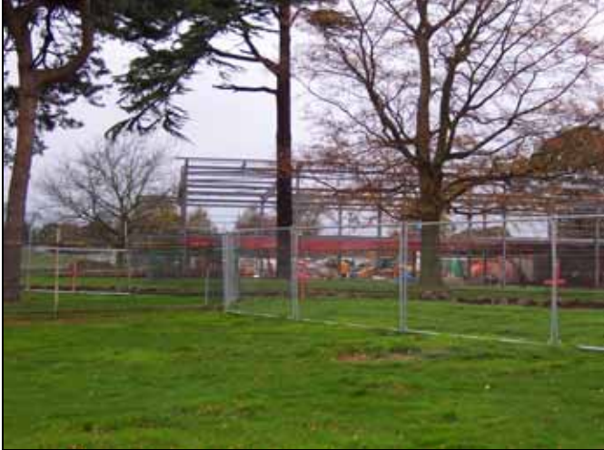
Construction work at Stoneleigh Business Park.
