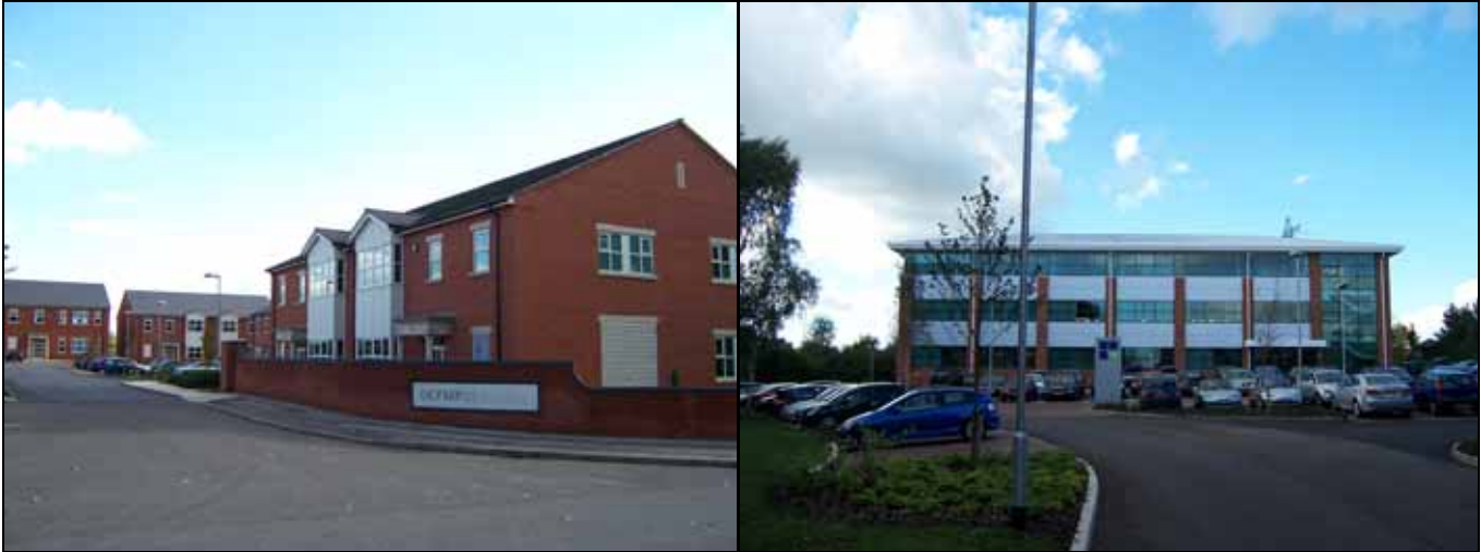
Office Development at Tachbrook Park completed during this monitoring year.
