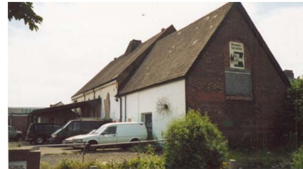
The Old School House No.16 Court Street offers scope to accommodate new uses within a refurbished building.
