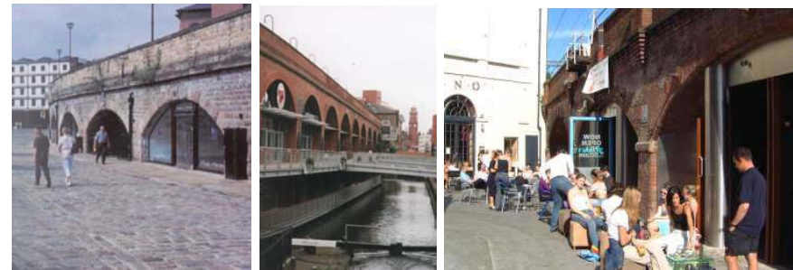
Creative reuse of railway arches is a real opportunity.
